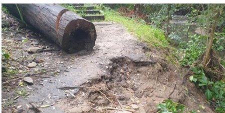
Increased water is causing bank erosion.
